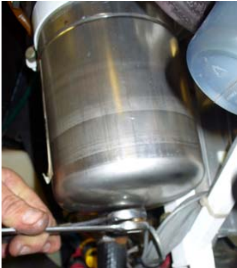
Figure 18: Undoing oil tank drain bung
