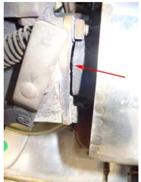
Figure 15: Crack in 914 exhaust pipe.
